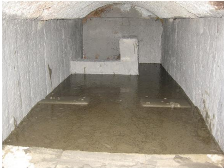
After Rehabilitation using Geopolymer grout
